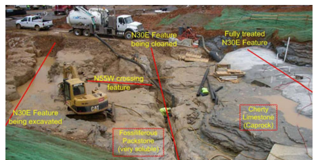
Fig. 5 Cleaning of N30E features
